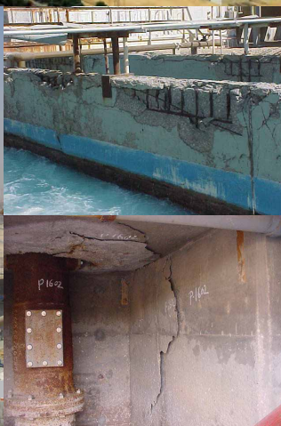
SEA WATER COOLING TOWER CONCRETE STRUCTURE
