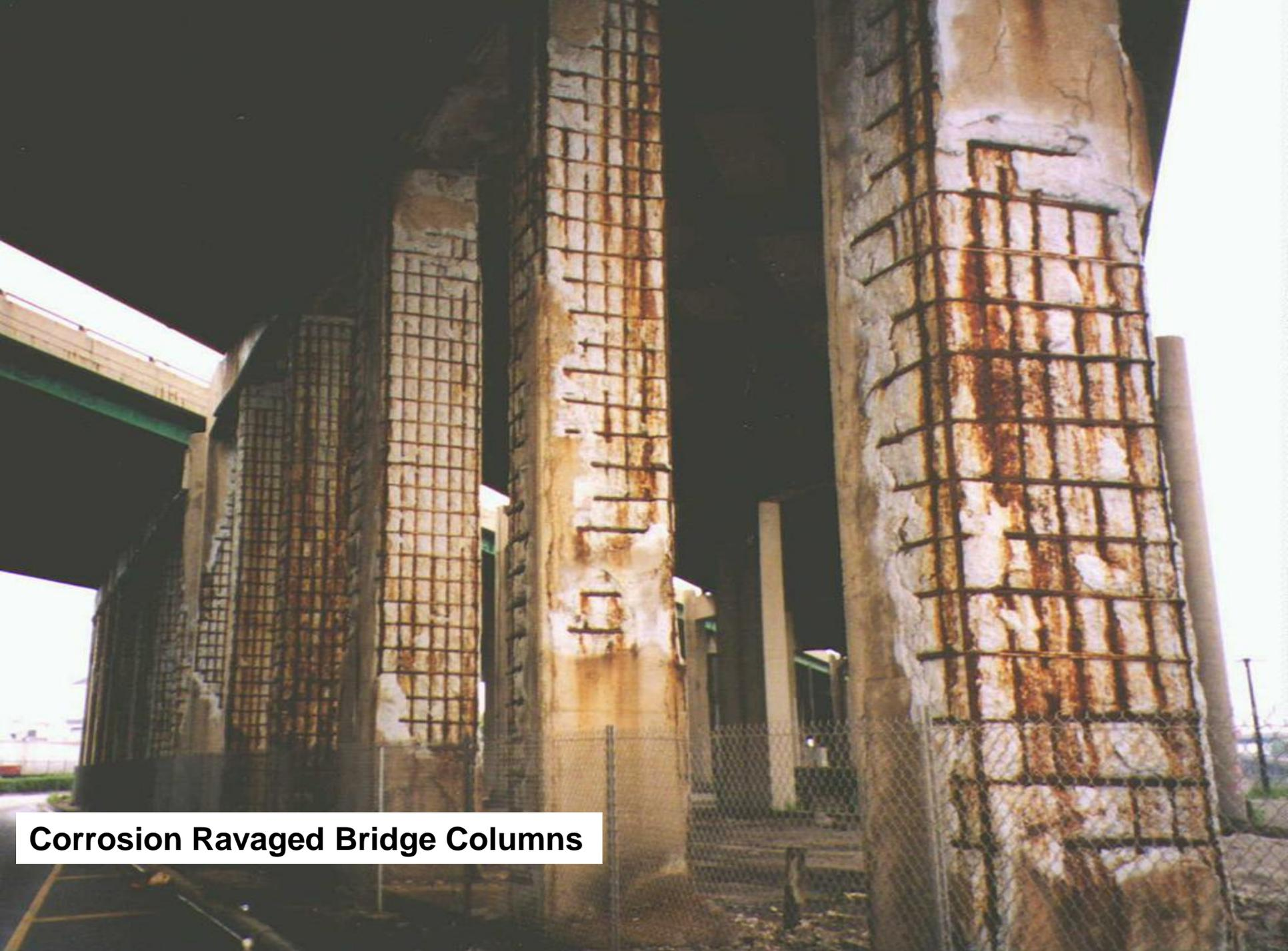
**Corrosion Ravaged Bridge Columns**
