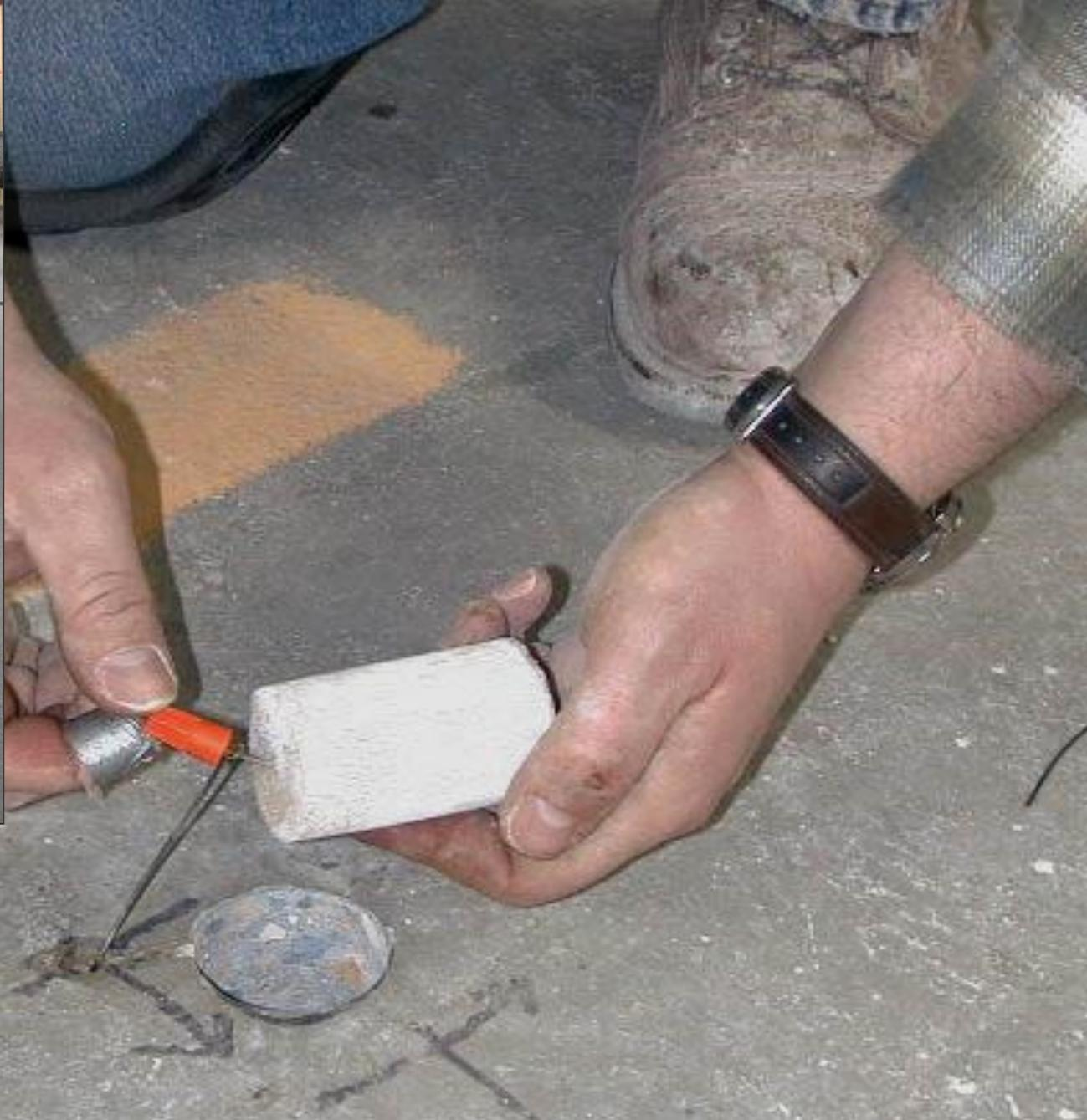
***Anode Connection to Reinforcing Steel***
