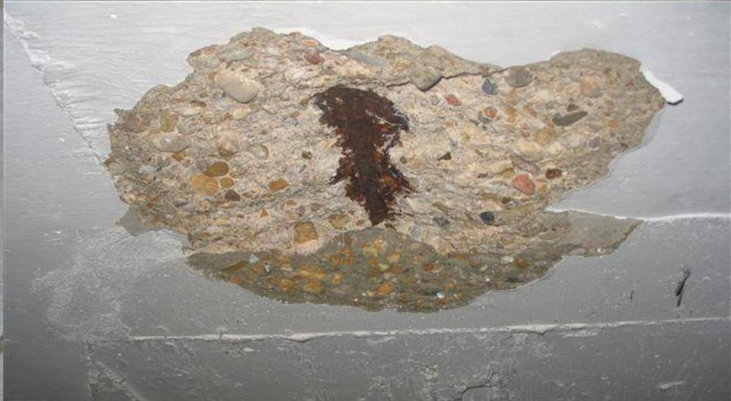
Halo Effect / Patch Accelerated Corrosion
