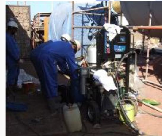
Dual Component Heated Airless Spray
