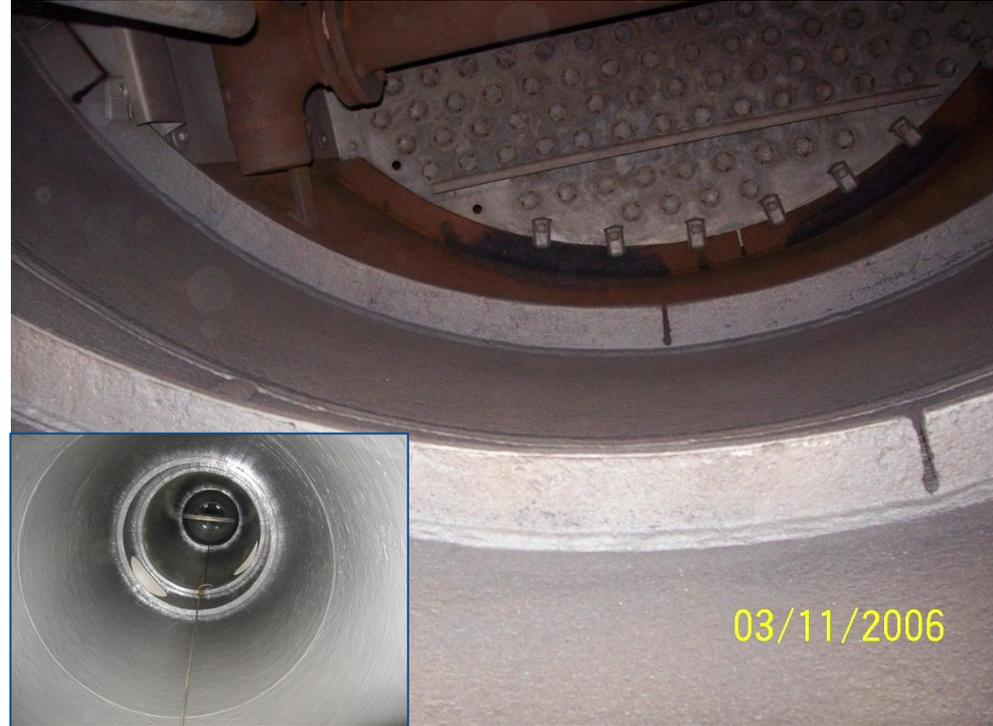
The acid washing process at elevated temperature led to severe pitting within the tower and significant loss of wall thickness adjacent to tray support rings. High Temperature repair compound used to restore wall thickness then acid resistant lining applied to resist operating conditions at 95C - Inspected in Year 2011 and in good condition.
