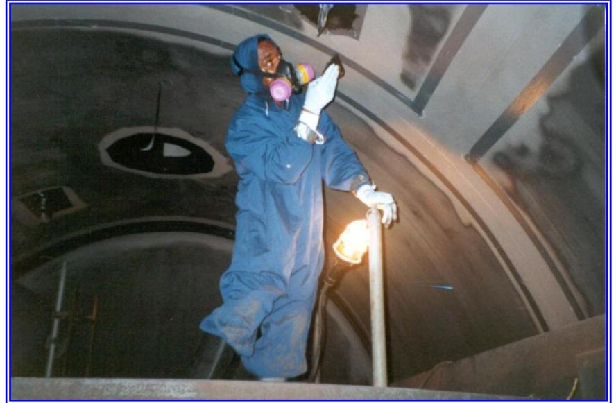
Protection of weld areas subject to stress corrosion cracking at elevated temperatures due to the presence of H<sub>2</sub>S. Weld areas only protected using high temperature Hybrid Epoxy Novolac lining system with operating temperature in excess of 150C
