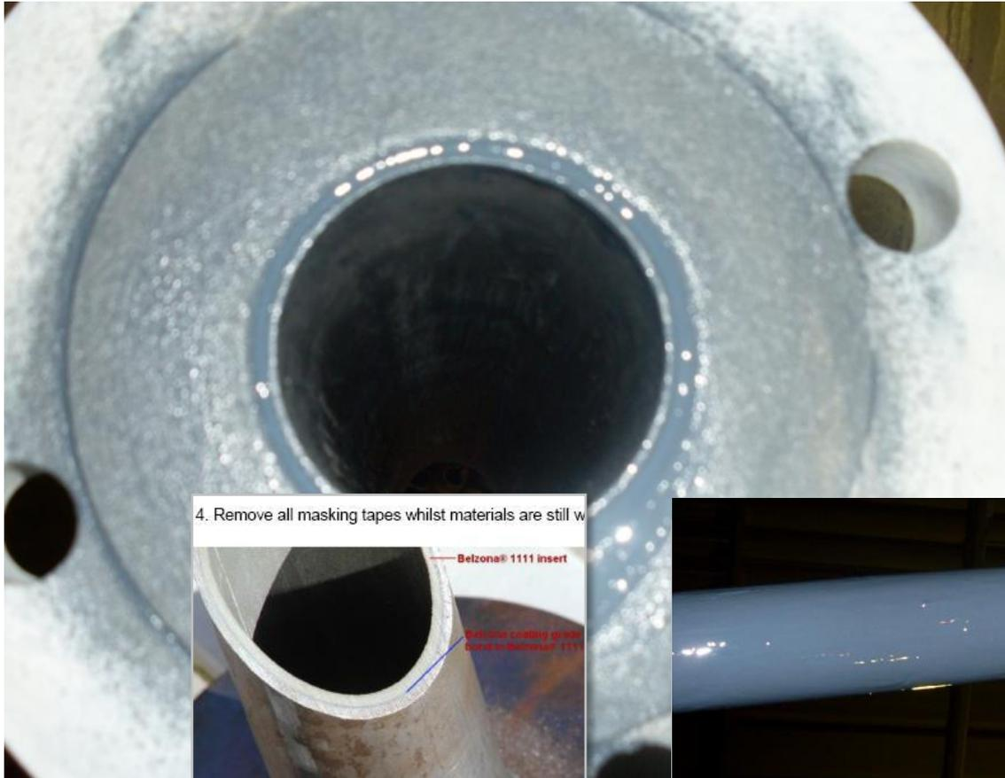
4. Remove all masking tapes whilst materials are still w
