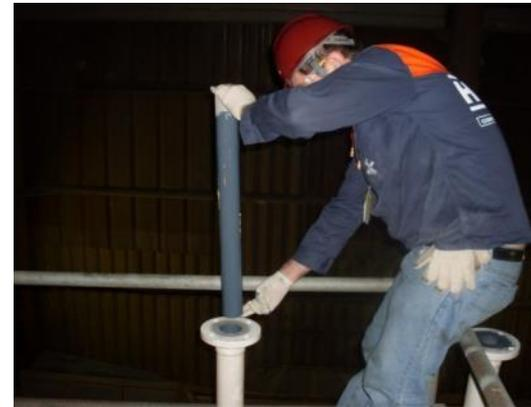
Belzona nozzle inserts bonded into small bore nozzles, protect against corrosion and erosion
