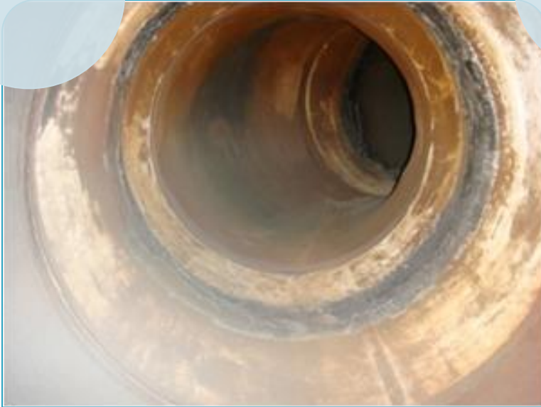
ENBBI, SAFANIYA WATER DISPSAL SYSTEM UPGRADE
